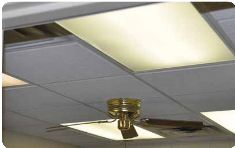
The new, energy efficient lighting (right) provides a much "whiter" light (measured in degrees Kelvin) than the traditional lighting (left). The co-op's switch will provide a payback of under 18 months, and will result in $4,956 savings on lighting costs annually.
